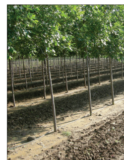
PE Tubing with On-Line Drippers in Nursery
