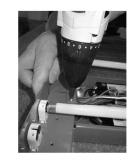
7. Remove the inner T5 lamps and begin adding the additional reflectors into place. Start from center portion of fixture and move outwards. Lastly, remove the outer T5 lamps and install the remaining two reflectors.
