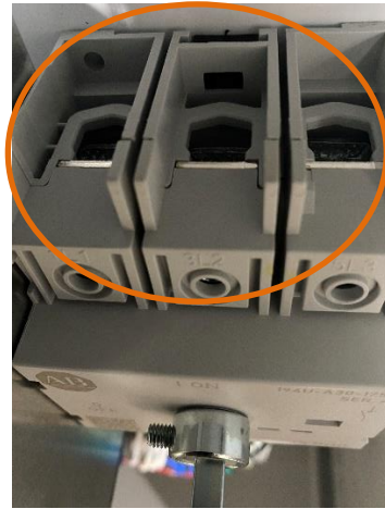
Figure 14: Input Terminal Connections on the Main Disconnect
