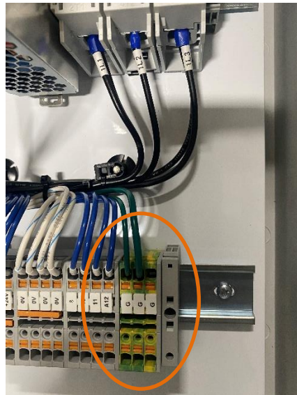
Figure 15: Shows the ground connection blocks.
